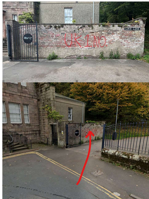
Site photographs: wall face (top) and location from Love Lane (bottom).
